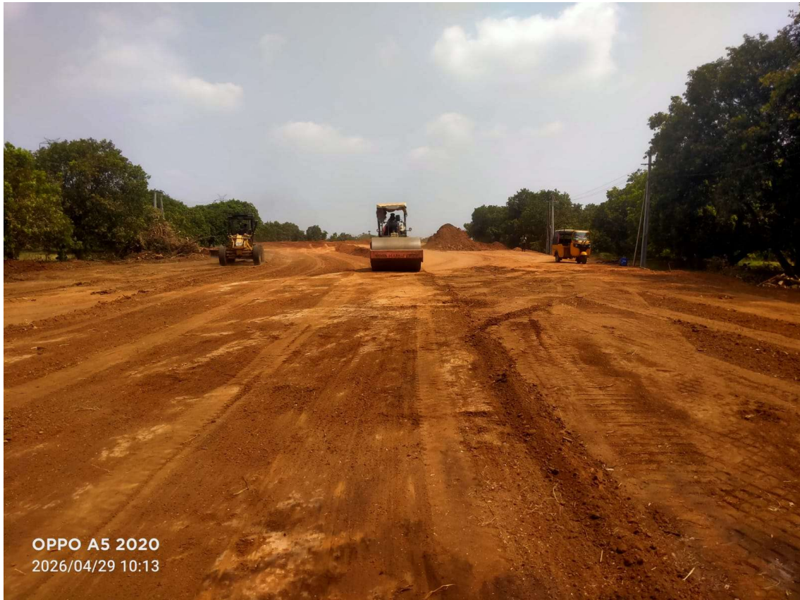
OGL bed rolling work in progress from 286+400 to 286+500 L/S
