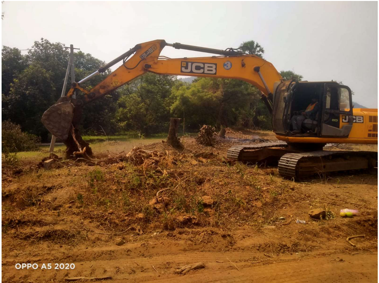
Mango stumps removing work in progress from ch 286+400 to 286+500 L/S
